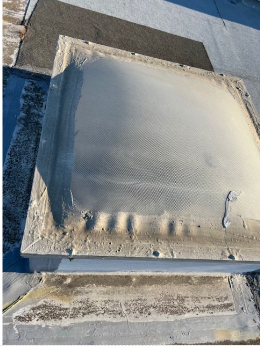
Skylight w/Sealant
