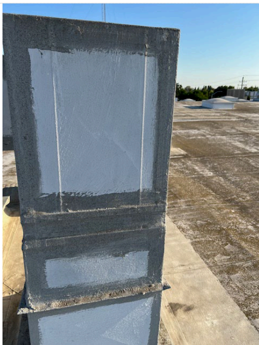
HVAC Ducts with Sealant
